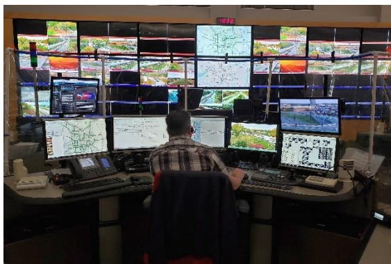
Figure 4: MnDOT RTMC Workstations with Clear Screen Curtains attached to PVC pipe Photo courtesy of MnDOT
